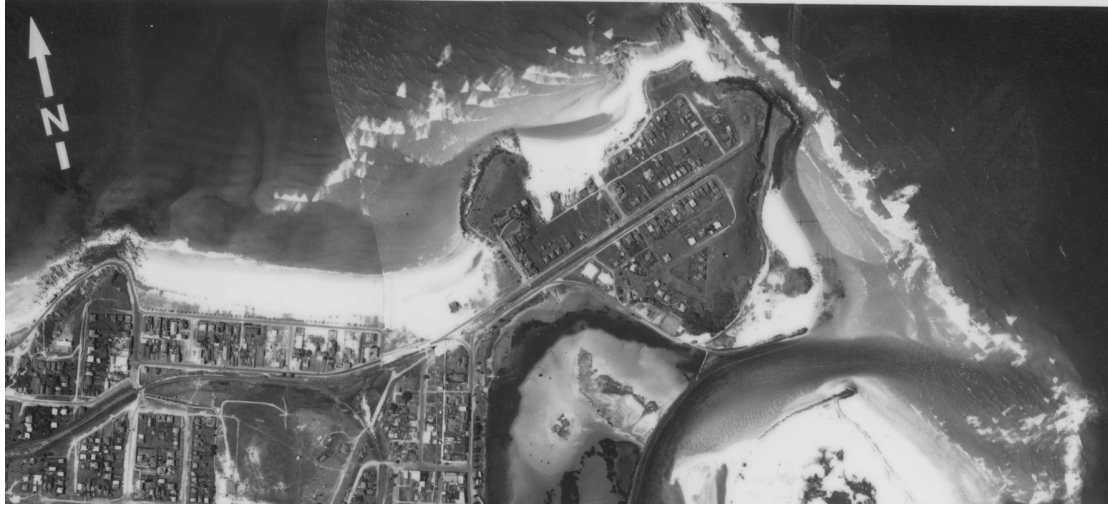
Figure 4 Point Danger and the Tweed River Entrance in 1935, before the Tweed River training walls were extended
